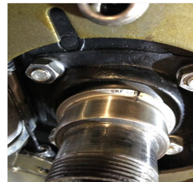
Sleeve fitted in the correct position with the ‘snipped’ collar ready for removal.
